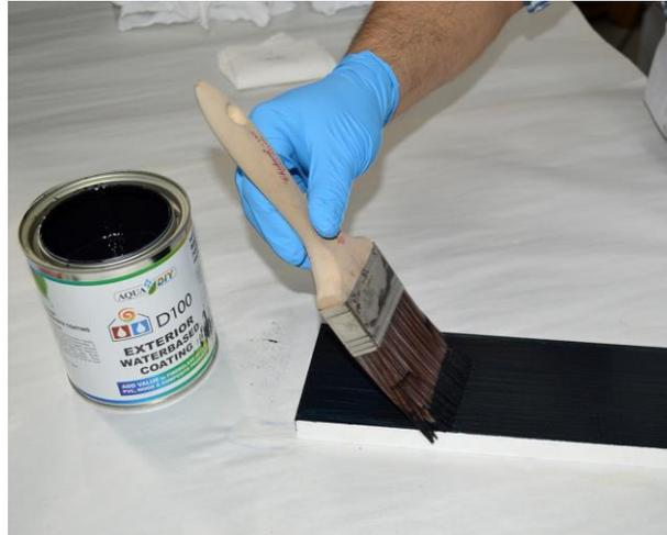
**For maximum efficiency, performance, and color quality, it is strongly recommended to perform a minimum of 2 even coats when brushing.**
